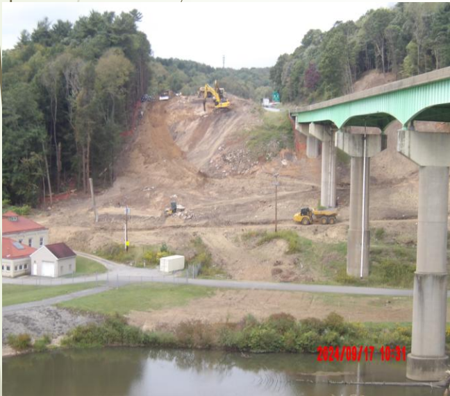
I-80 Bridge Project, Brookville Borough & Pine Creek Township
