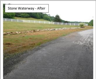
**Problem:** An existing stone lined ditch could not carry heavy rain events and flooded the Borough Road. Existing pipes along the Borough Road transitioned from a 24" pipe down to a 15' pipe, causing repeated flooding. Repeated flooding caused severe erosion around the outlet of an undersized cross pipe.
