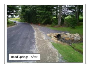
**Problem:** The road base was saturated by water coming from two road side springs and a pond located directly along the road. There was flowing water in the existing ditch.
