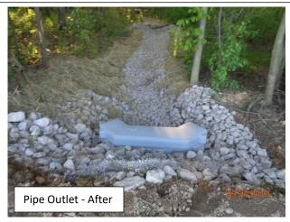
**Problem:** A large amount of stormwater was concentrating between two Township roads, causing a severely eroded gully to form. Existing crosspipes were too small. The outlets of the existing crosspipes were failing, causing the surrounding banks to erode.
