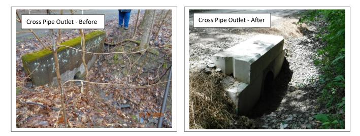
**Problem:** The existing cross pipes were too small. The existing end walls were crumbling and falling into the outlets. Erosion was occurring at the outlets of the existing cross pipes. Some of the inlets needed stabilized.
