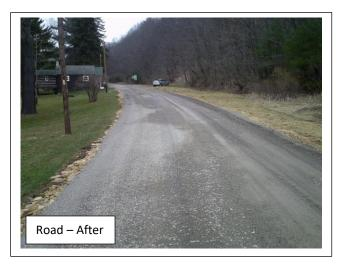
**Problem:** Water from the hillside was saturating the road base. Road was flat and ditch full of water. The road surface was full of potholes. The existing crosspipe was too small.
