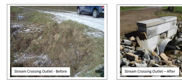
**Problem:** The existing stream crossing had double pipes and they were too small, which caused erosion on the surrounding streambanks. Water was running very long distances in the road ditches, carrying sediment directly to the stream.
