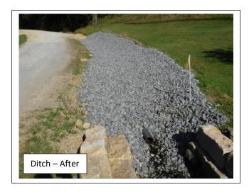
**Problem:** Roadside springs were saturating the existing road ditches. Water was laying in the ditches saturating the road base. There was a limited number of existing cross pipes and they were too small.
