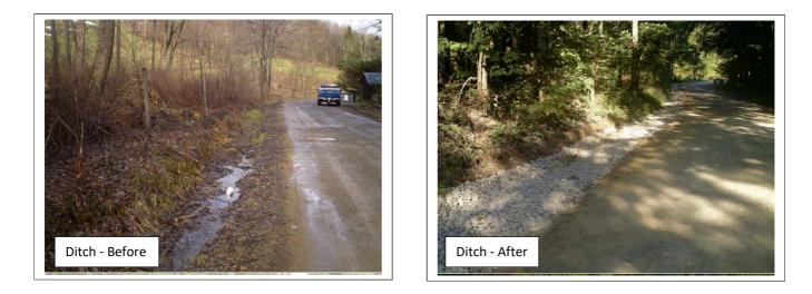
**Problem:** A roadside spring flowed into the road ditch, causing the it to become saturated and the road base to sink. A small stream discharged into the road ditch and flowed in two different directions, adding additional flow and saturation to the ditches. Existing cross pipes were undersized.
