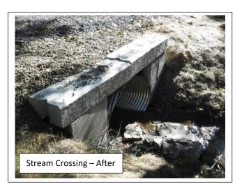
**Problem:** The existing stream crossing was too small, which caused erosion on the streambanks and stream bed. Water was running in the road ditch for a long stretch, causing deep ditches. The road was entrenched.
