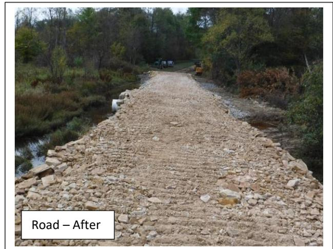
**Problem:** Wetlands are on both sides of the road. Water from one side occasionally overtopped the road, which caused erosion and carried sediment into the wetland on the opposite side. The elevation of an existing overflow pipe was too high and was in an unfavorable location.
