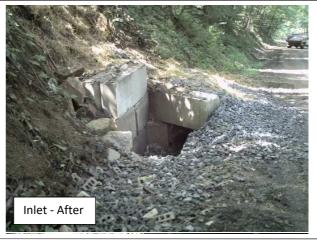
**Problem:** Road banks were eroding into the existing cross pipe inlets. There were roadside springs. There was erosion at the outlets of cross pipes and steep banks. Water was running from springs, coming out of the nearby hillside, flowing along the Township road. This caused the flow in the existing ditch to begin undercutting the road.
