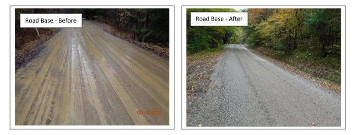
**Problem:** The existing cross pipes were undersized, and some were collapsing. There were no head or end walls on the cross pipes. The road base was soft and flat.
