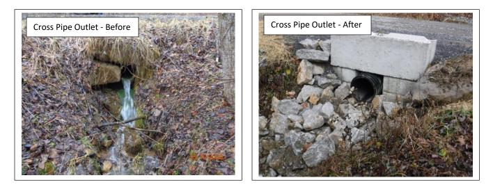
**Problem:** The existing cross pipes were too small, causing erosion at the outlet of the pipes. Standing water in some of the roadside ditches was causing water to saturate the road base, creating potholes. The lack of head and end walls on the existing cross pipe was causing the road bank to erode.
