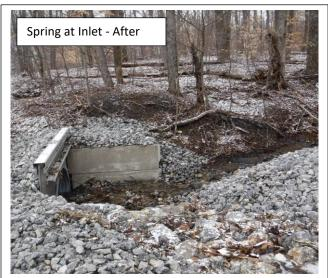
**Problem:** A continuous flow of water from numerous roadside springs and an extended length of paved road ditch. The existing cross pipe was severely undersized and a portion of it was filled with debris. The bottom of the existing cross pipe had completely eroded away. The outlet of the existing pipe was perched and was causing severe erosion.
