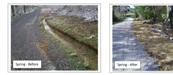
**Problem:** An underground spring was discharging directly into the road base, causing it to become saturated. An existing cross pipe had collapsed. The road profile was not crowned.
