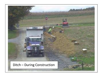
**Problem:** Underground springs were leaching out of the road bank and flowing into the existing road ditch. A field drain also discharged into the existing road ditch. The road profile was low and causing the road to act as a ditch, carrying sediment directly to the stream. Severe erosion occurred in the ditch due to several large rain events.
