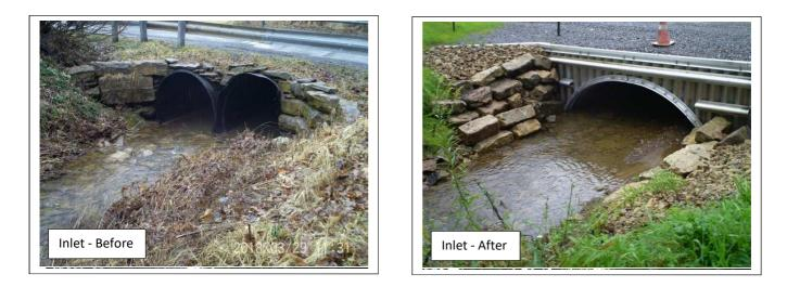
**Problem:** Water from a roadside spring was carrying sediment directly to the stream. The existing twin plastic pipes that had been joined to a cement box culvert were separating, causing the road to begin to collapse. The twin pipes were causing erosion along the stream banks from the water backup.
