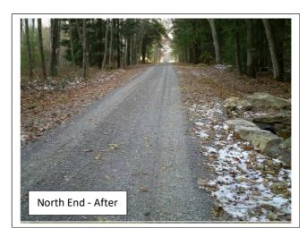
**Problem:** There was a roadside spring running along the road. The existing underdrain was plugged. Offsite runoff was entering the roadway from a camp's driveway. The road grade was lower than the surrounding area. The road was acting as a ditch and was carrying sediment directly to the stream. A field drain discharged water along the road.
