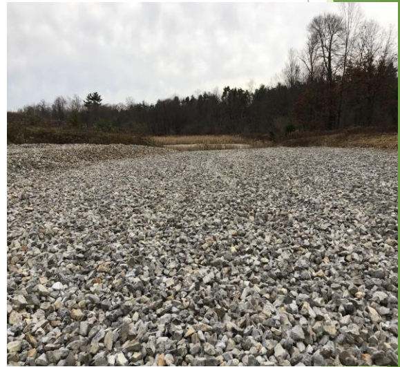
Limestone bed with subsurface drainage
