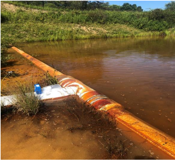
Manifold and pooled water
