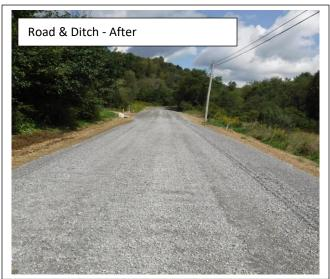
**Problem:** Excessive runoff in a long length of road ditch that also discharged directly to a stream. The saturated ditch along with springs along the road caused the base to become soft.
