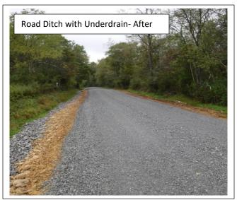
**Problem:** Lack of adequate cross pipes and saturated road ditches cause the road to become soft.
