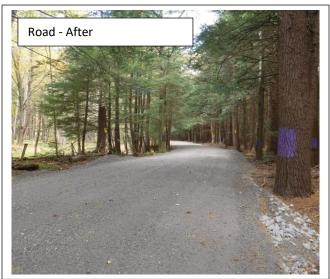
**Problem:** An inadequate cross pipe and a poor road profile caused surface flow onto the roadway during rain events.
