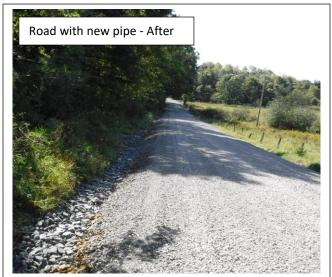
**Problem:** An entrenched road down a steep grade had excessive runoff on both sides during rain events. Additional runoff entered the roadway from an adjacent access road. 2 existing cross pipes discharged at the same location.
