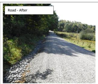
**Problem:** 3 roadside springs were saturated road ditches, with constant flow causing them to cut deeper, conveying sediment directly to the nearby stream. This saturation was also causing the road base to become unstable.
