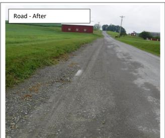
**Problem:** An existing 12" cross pipe was inadequate to convey runoff from the road ditch and an adjacent pond overflow.
