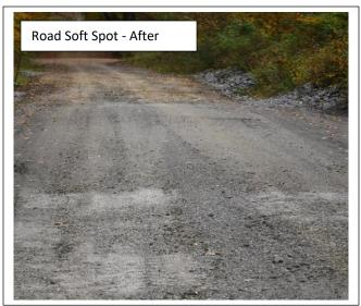
**Problem:** Large amount of runoff being conveyed down a steep grade in an excessively deep ditch. A spring located in the roadway. The entrenched road provided no option to outlet the runoff, causing the road ditch and road base to become saturated. An existing cross pipe was inadequate during rain events.
