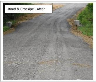
**Problem:** Two roadside springs were overwhelming an existing cross pipe. One roadside spring was saturating the existing ditch, road base and flowing across the Township Road. This caused the road and the road base to become soft. Sediment was being conveyed in the road ditches during rain events.
