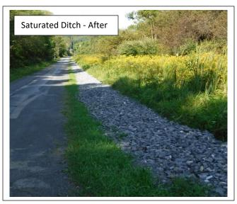
**Problem:** Existing ditches were saturated with groundwater, causing road base cracking.
