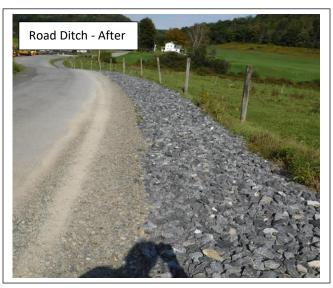
**Problem:** Runoff from an existing Penn Dot cross pipe and a spring located in the middle of the Township Road were saturating the Township Road ditch with flowing water. Sediment was being conveyed directly to the stream.
