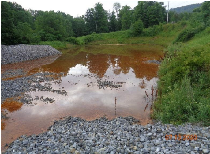
Standing water prior to maintenance
