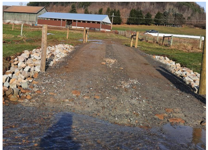
After- stabilized livestock stream crossing
