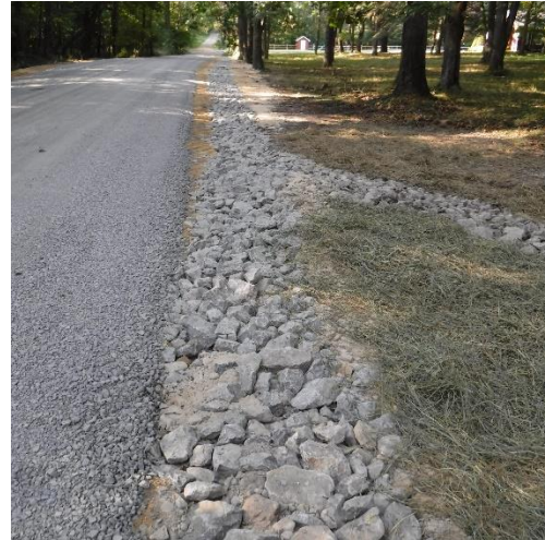
A severely eroded ditch and washed-out roadway was repaired by building up the roadway 3 to 4 feet, installing 2 tear drop filtration systems, a new stone lined channel.
