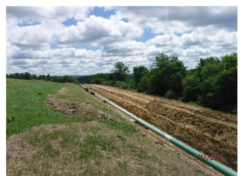
Brockway Modernization, Brockway
