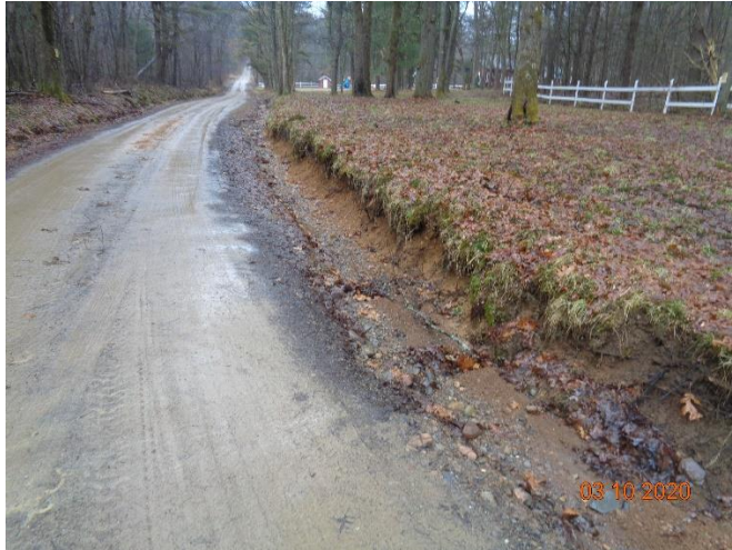
A severely eroded ditch and washed-out roadway was repaired by building up the roadway 3 to 4 feet, installing 2 tear drop filtration systems, a new stone lined channel.
