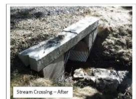
Stream Crossing - After
