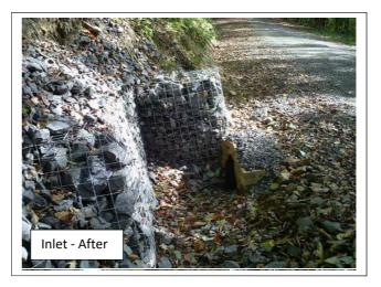
**Problem:** The road bank was eroding into the inlets of the existing cross pipes. There were not enough cross pipes. The existing road profile was lower than the surrounding area and did not contain a crown. The road was acting as a ditch. The existing ditches were too deep.
