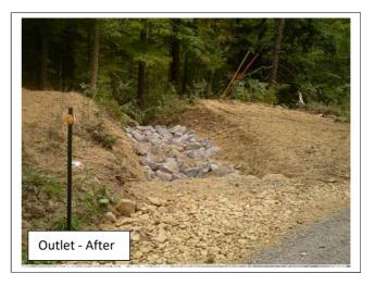
**Problem:** Runoff had to travel a long distance in the road ditch before entering existing cross pipes. The existing cross pipes were undersized and could not handle the runoff from heavy rain events. Runoff overflowed at the cross pipes, causing erosion on the road and at the cross pipe outlets. An outlet from an existing field drain was directed into the road ditch, causing erosion and increased runoff in the ditch.
