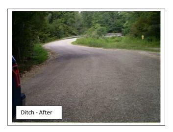
**Problem:** A road side spring, groundwater and a lack of cross pipes were causing the road base and the road ditch to become saturated.
