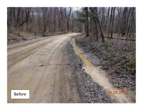
**Problem**: Due to wetlands on both sides of the road and poor drainage, the road base was saturated. An existing cross pipe was plugged and crushed.
