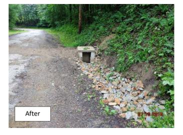
**Problem**: Excessive stormwater was running down the long, sloping road. Ditches were eroding and overflowing, existing cross pipes were not sufficient. The runoff was concentrated to one area, causing severe erosion.
