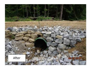
**Problem**: Stormwater from an adjacent Penn DOT Road was being directed onto the Township Road, causing severe erosion. The Township Road was acting like a ditch, conveying sediment laden runoff directly to the stream. Existing springs along the Township Road also contribute to make a soft road base. The existing stream crossing was undersized.
