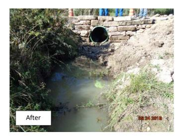
**Problem**: Stormwater runoff was entering the entrenched roadway from an adjoining driveway as well as the top of the hill. Since runoff cannot leave the roadway, erosion is occurring and sediment is going into the nearby stream. The existing stream crossing is collapsing and is not functioning properly. The road profile was very flat.
