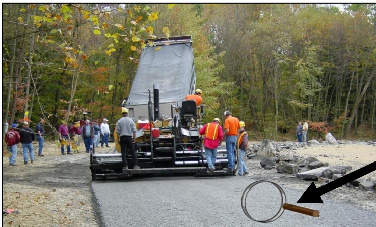
Figure 1: Placement of DSA through a paver.
