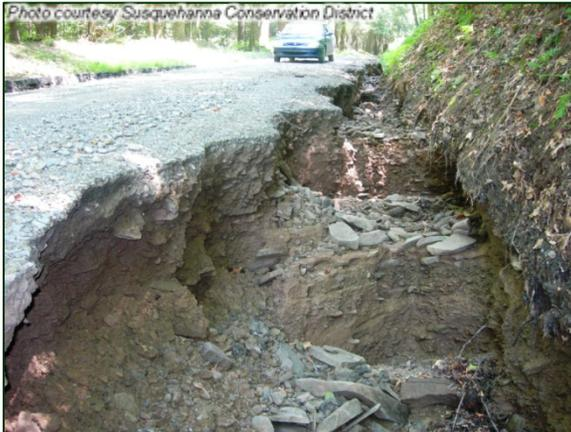
*A badly eroded ditch on its way to a nearby stream*
