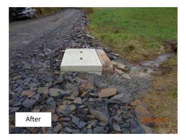
**Problem**: Ponds on each side of the Township Road were discharging onto the road, saturating ditches and the road base. The road was entrenched, acting like a ditch, picking up water from the top of the hill.
