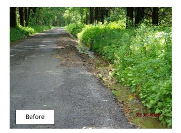
**Problem**: Water from several sections of Songer Road was being directed onto Shaffer Road, where it was washing out the ditches and eroding the existing driving surface.
