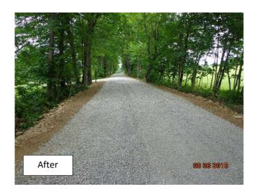
**Problem**: The Township Road was entrenched, acting as a funnel for a large nearby field. The concentrated runoff repeatedly washed out the ditches, directing sediment to the nearby stream.
