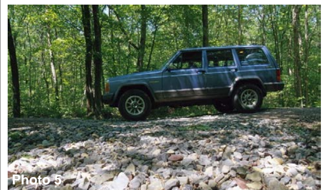
Finished bypass blends into rest of road.
