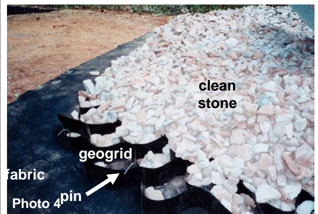
Fabric, geogrid, and #3* stone.
