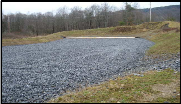
Conifer Treatment System FeAlMn bed
