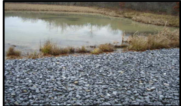
Treatment System outfall
