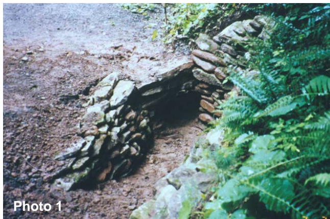
Headwall at pipe inlet.
